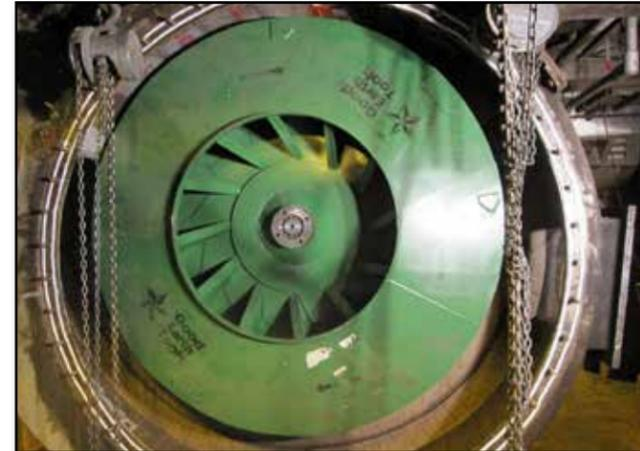
A GET high efficiency Carbide fan is installed and ready to roll at this power plant. Carbide wear protection will keep it in service for years.
